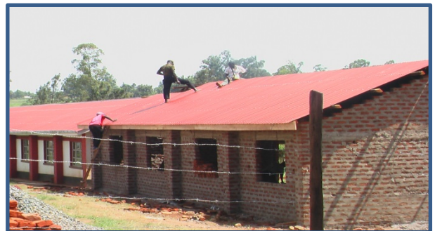
Laying Iron sheets on the back phase
