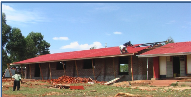
Laying iron sheets on the front phase
